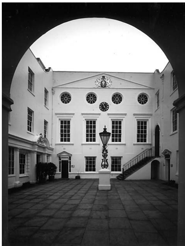
Figure 3 The courtyard of Apothecaries' Hall, Black Friars Lane, London.
